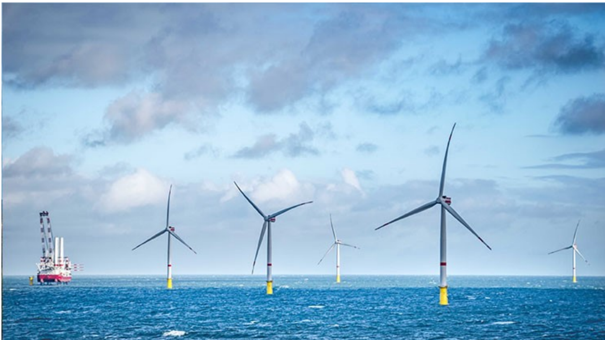
Figure 1: Vineyard Wind Farm, Massachusetts. Courtesy of Iberdrola.
